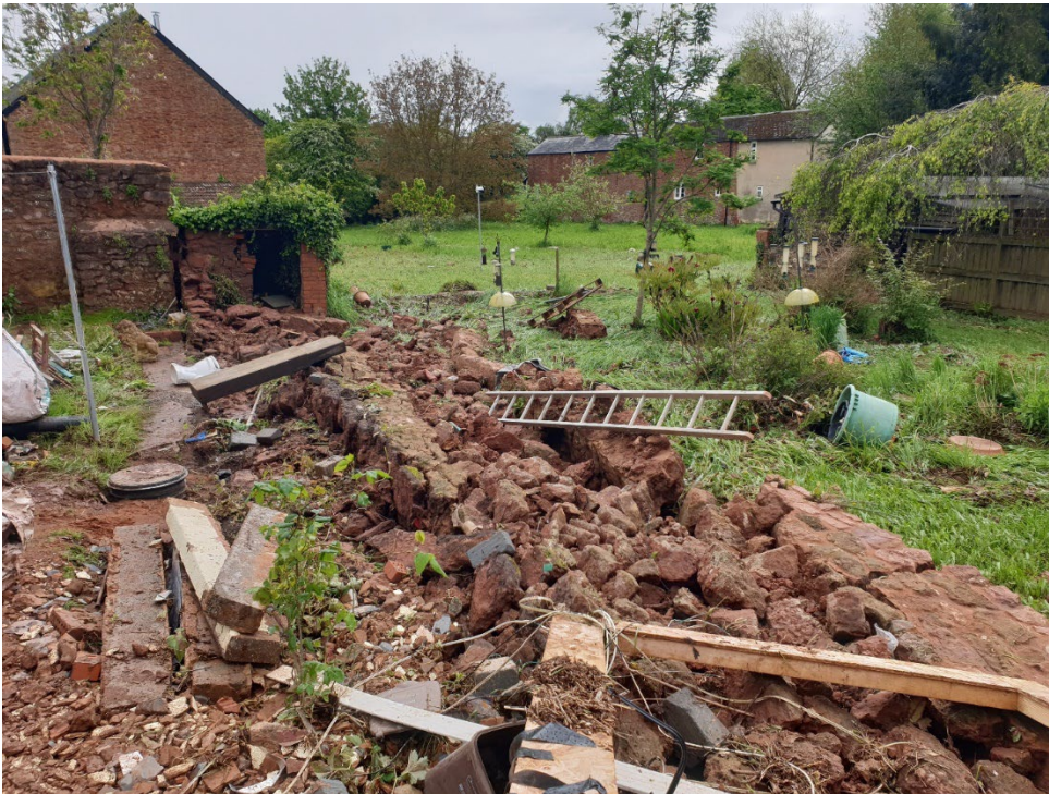
Figure 1. Flood Damage, Milverton, May 2023
